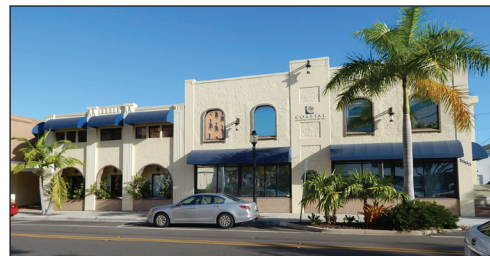
1565 State St., Sarasota – SALE PENDING 12,655 gross square-foot office building, 15,750 square feet of land, zoned DTC. $2,700,000
